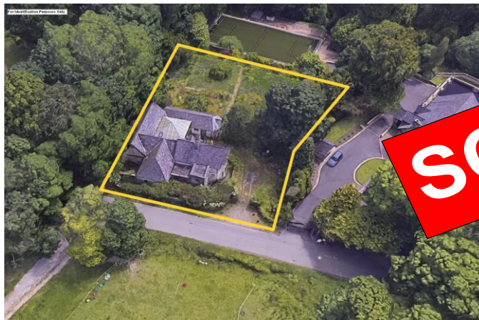
Ousel Nest Gatehouse, Grange Road, Bromley Cross, Bolton BL7 9AX
